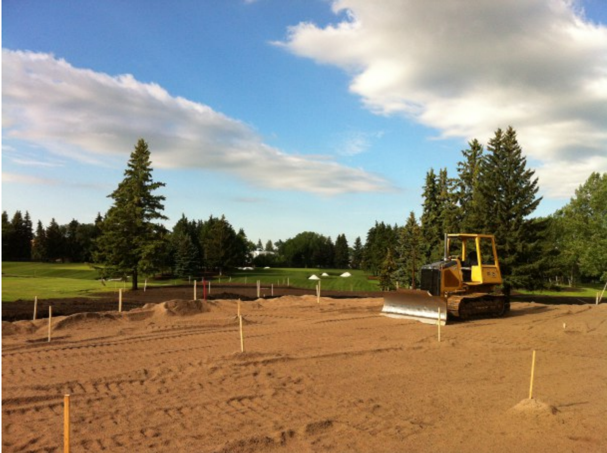
The first hole, under construction.
