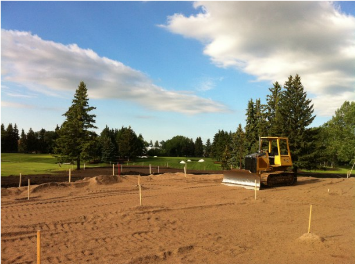
The first hole, under construction.
