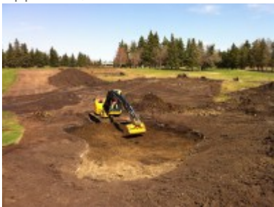
George, shaping a bunker
