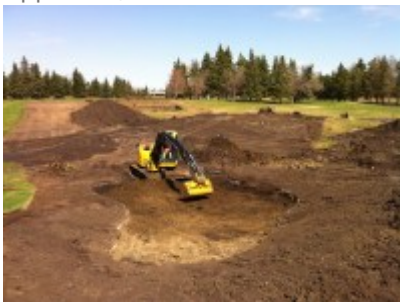
George, shaping a bunker
